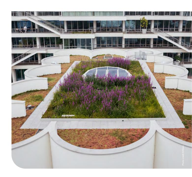
Skywater Clear is an innovative system of treating grey water by roof-based constructed wetlands designed in collaboration with Aquatiris, the French leader in constructed wetlands engineering, and is the only solution of its kind in the world.
